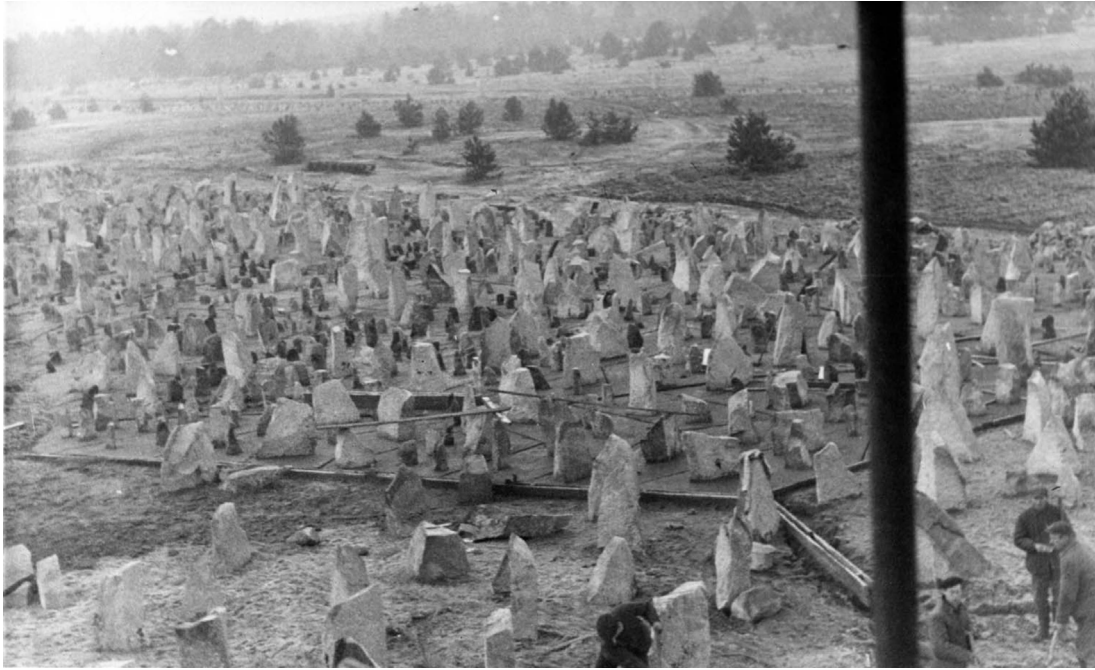
Consecutive stages of the work photographed in 1963, probably by Adam Haupt. In the foreground the concrete is about to be poured. Right behind this, the concrete slab is ready (Photograph from Adam Haupt's archive, cited after: Radecka, 2011)
